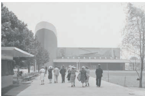
Lyonel Feininger, Marine Transportation Building, New York World's Fair 1939/40, 1939 . Private collection. Image courtesy of Moeller Fine Art Projects. The Lyonel Feininger Project, New York-Berlin.
